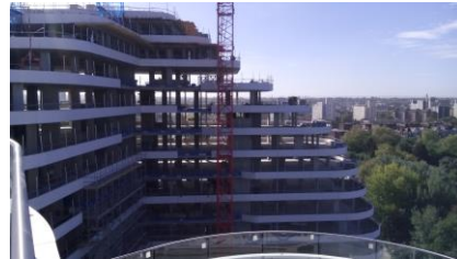
Block L –Concrete frame is complete.
