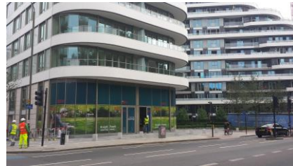
Block C – Core 1 is now complete.
