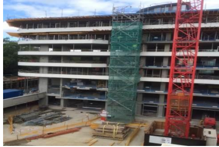
Block C has progressed on to the seventh floor on Cores 1 & 2
