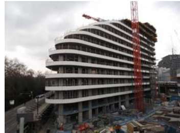
Block C is now at Level 15 and the roof has been cast.
