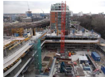
Block L is progressing and is at Level 4.
