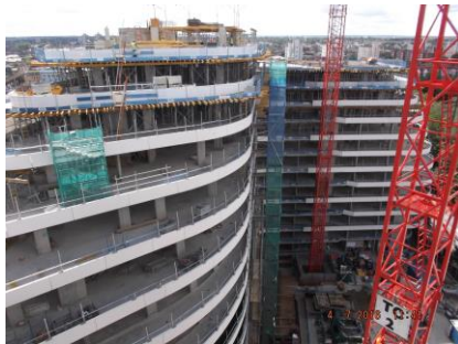
Block L is progressing and is at Level 6.
