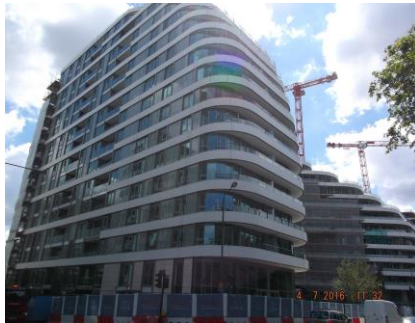
Block C – The concrete superstructure is now complete
