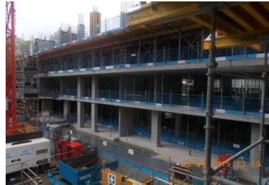
Block C has progressed on to the second floor on cores 1 & 2
