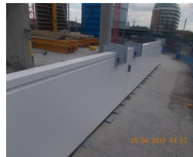
Balcony panel installation has commenced on Block C
