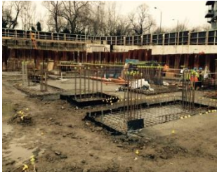
Ground works are progressing on the north elevation, with most of the pile caps completed on Block-C
