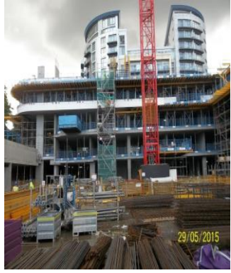
Block C has progressed on to the third floor on cores 1 & 2
