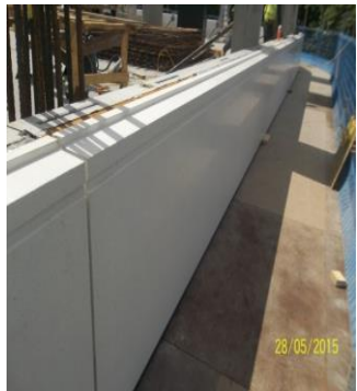
installation has been completed on levels 2 & 3
