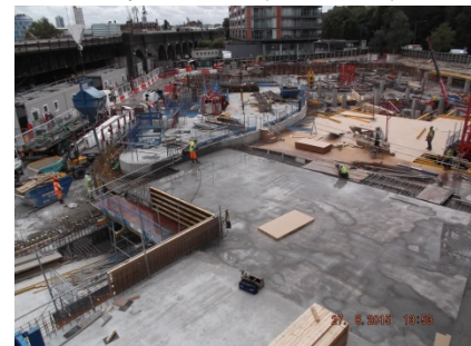
Progress is ongoing on the podium slab along the Car Park Section.
