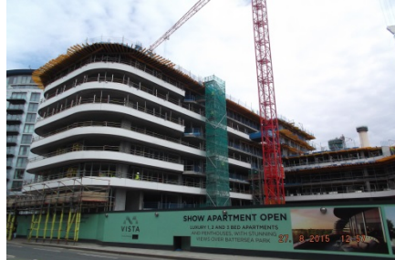
Block C has progressed on to the 8 th floor on Cores 1 & 2
