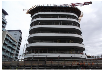
Balcony panel installation is progressing and currently on Level 8 (cores 1 & 2)
