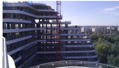
Block L –Concrete frame is complete.
