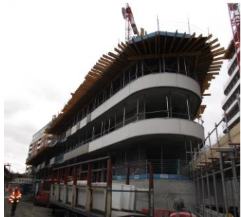
Block L is progressing and is at level 2.
