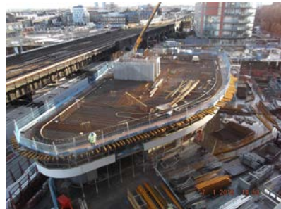
Block L is progressing and is at level 2.
