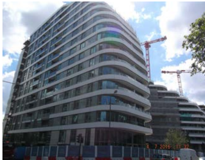
Block C – Core 1 is now complete.
