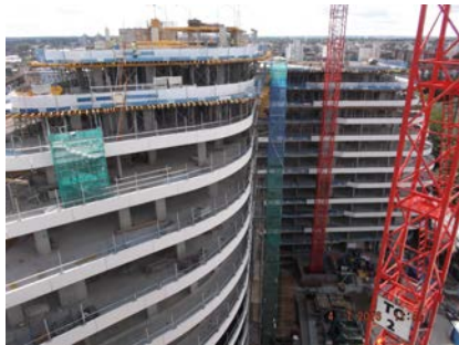
Block L is progressing and is at Level 14.
