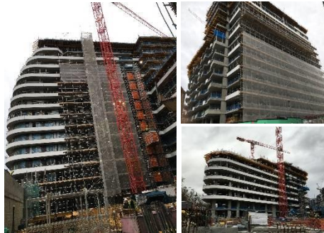
Block C has progressed to the 14 th floor (cores 1&2)
